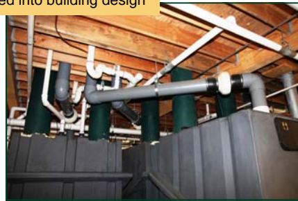
Composting system is integrated into building design
