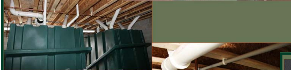
Men's composter with 2 foam-flush toilet pipes, 2 urinal lines, and vent pipe
